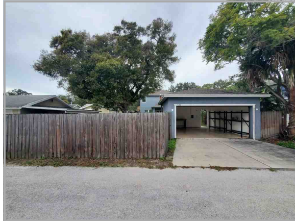
Rear View from Alley
